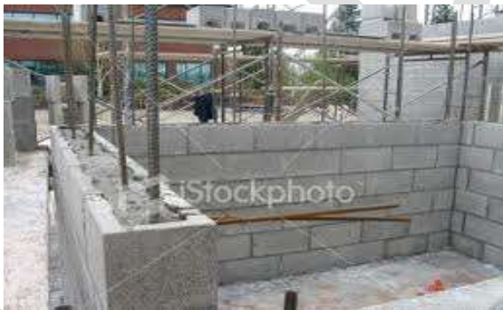
Fig 3: Concrete block walling
