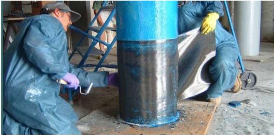
Fig.1.1.Jacketing of GFRP sheets around column
