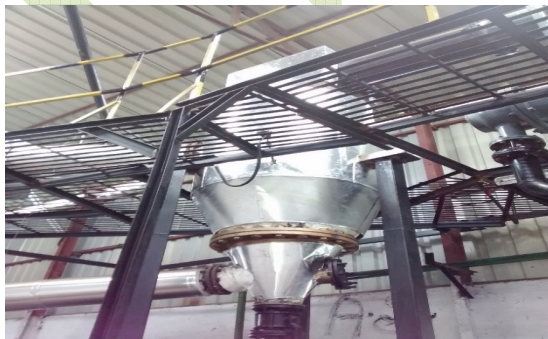
Figure 5: Cyclone Separator
