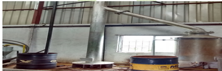
Figure 8: Pressure Controlling System
