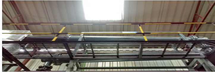
Figure 7: Condenser and Receiver assembly
